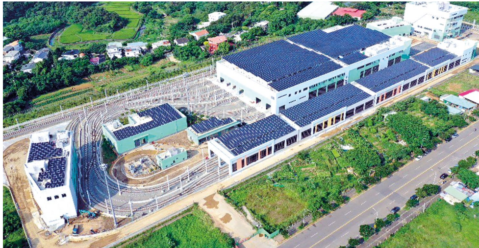
Solar PV system at Danshui Light Rail Machine Factory
